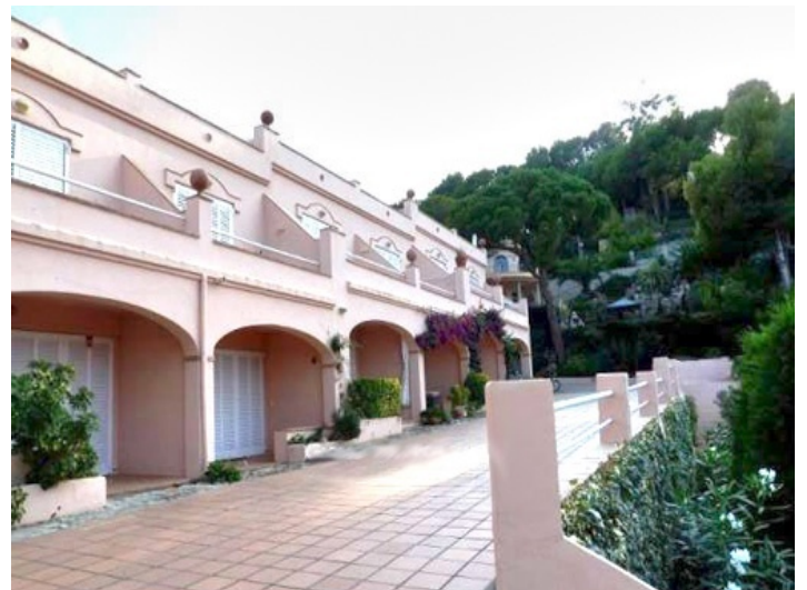
Front view with porch
